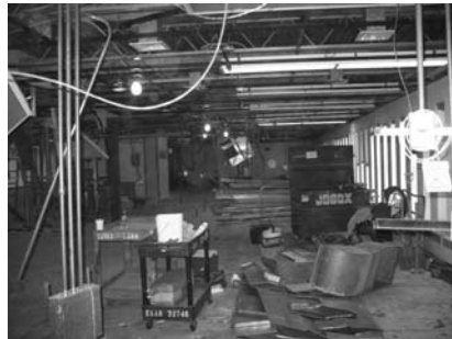
Old administrative offices
